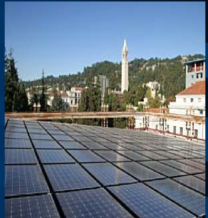
UC Berkeley's 120 kW PV array, located on Martin Luther King Student Center roof
